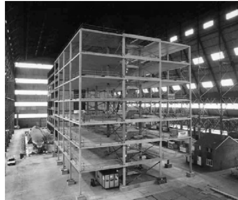
Figure 1. A multi-panel concrete building used in the research work (after ICE, 2000)
