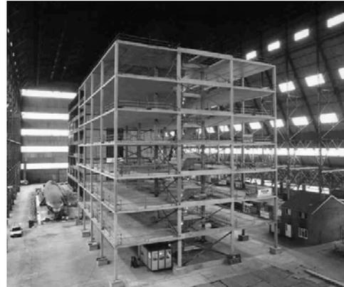
Figure 1. A multi-panel concrete building used in the research work (after ICE, 2000)
