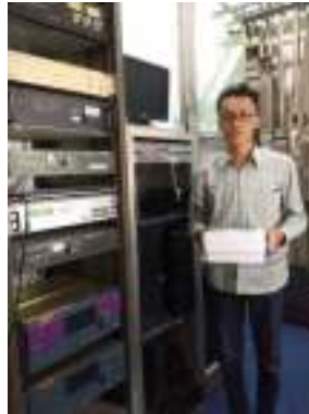
Gambar 10. Potret Ruang Server LPP RRI
