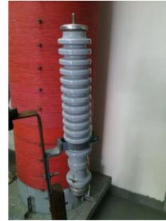
Gambar 6 *Lightning Arrester* tipe SiC
