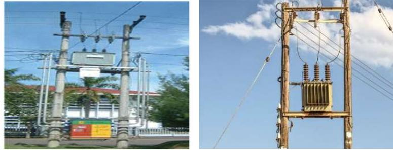
Gambar 1. Transformator jaringan distribusi 20 kv
